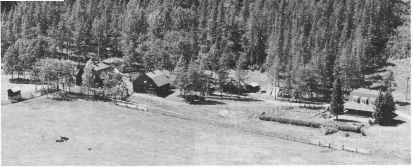
Connop's Bar Twin Cee Ranch. House and barns built in 1925, replacing original buildings. 1962 photo.
